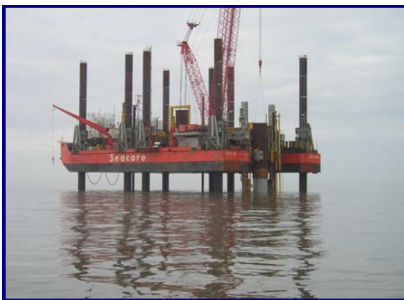
Hammer piling wind turbine foundations generates significant underwater noise.
